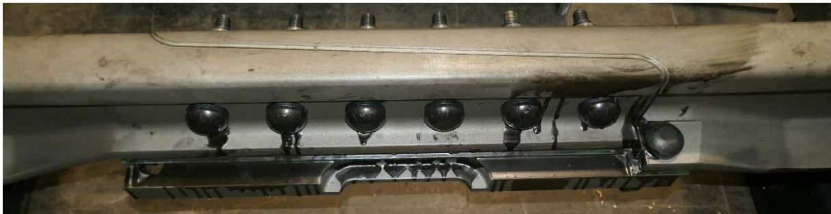
Figure 2: Opposite view of insulated joint "ABJ"
